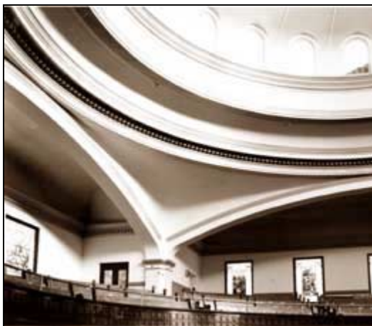
Plaster was used as the interior surface coating of this
